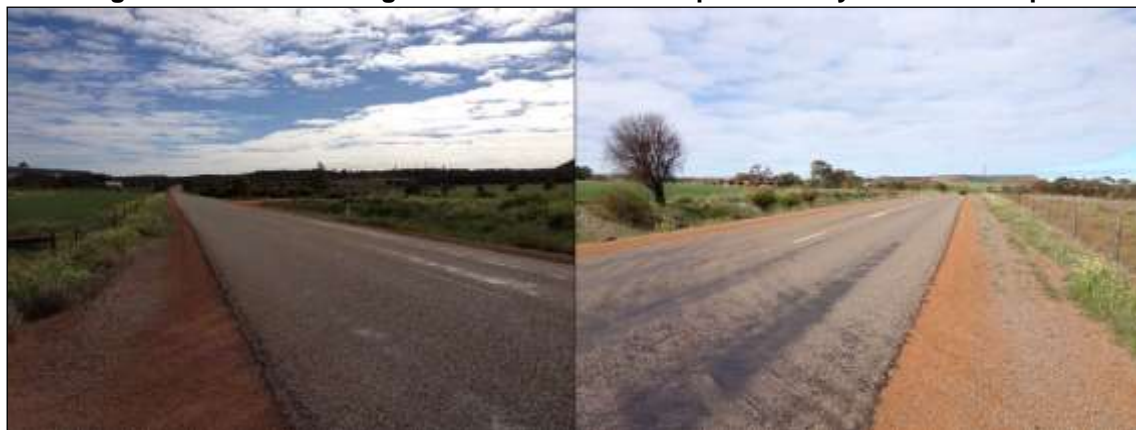
Figure 5 – Views looking north and south at Chapman Valley Road access point
