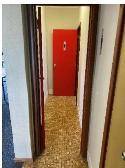
Narrow airlock (600mm) to upstairs function room toilets, No accessible facilities
