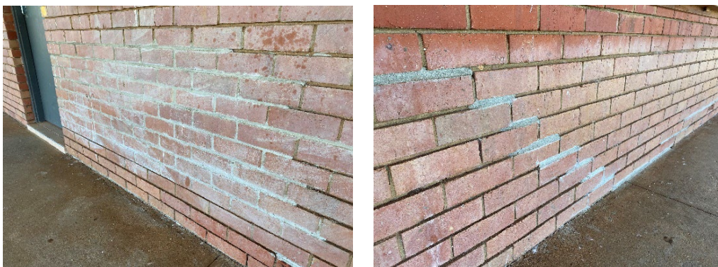
Mortar repairs, brick movement
