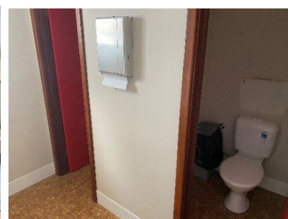
Narrow airlock (600mm) to upstairs function room toilets, No accessible facilities
