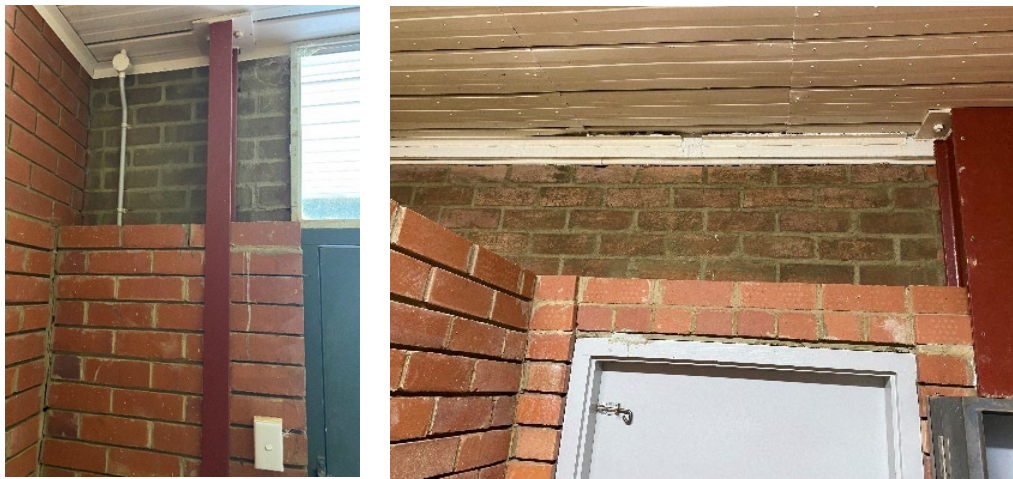
Incomplete double brick work
