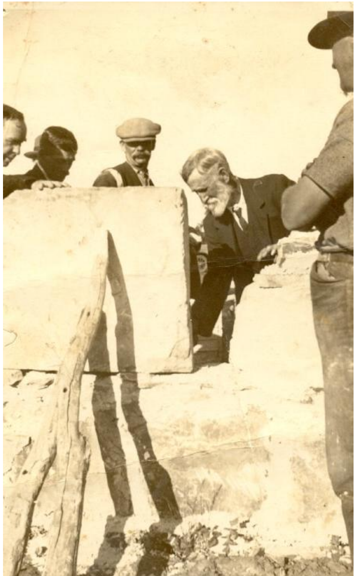
James Criddle Laying Foundation stone
