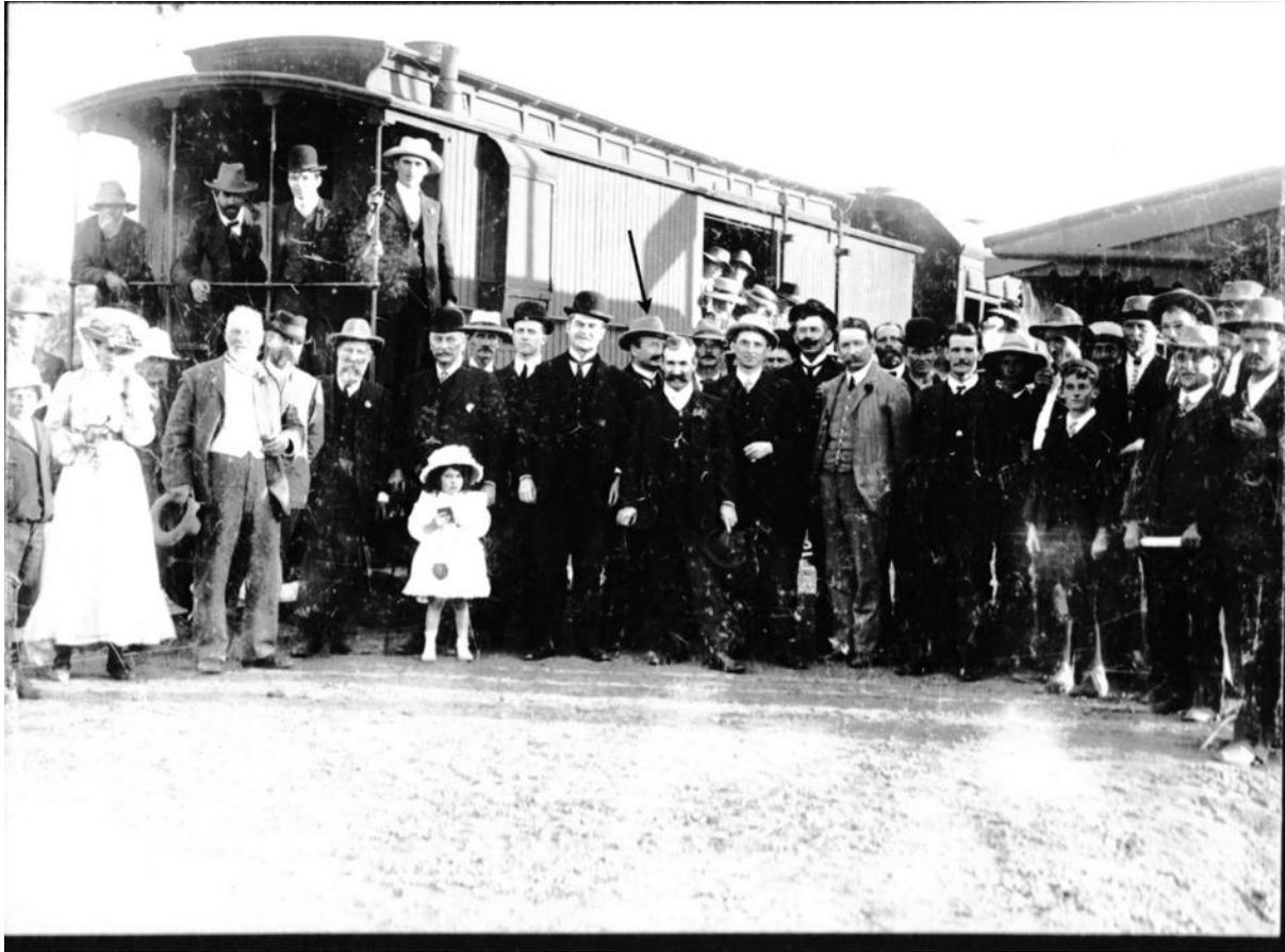
Naraling Railway Siding opening Arrow: Contractor Richard Rennie
