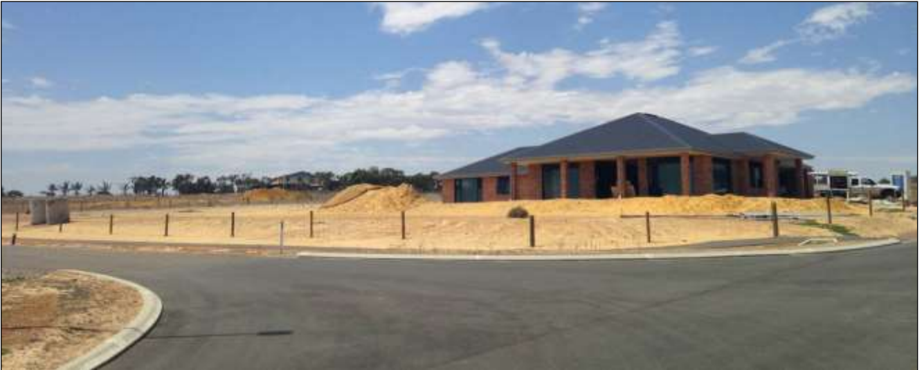
Figure 4 – View looking north-east from Hilltop Loop towards Lot 118
