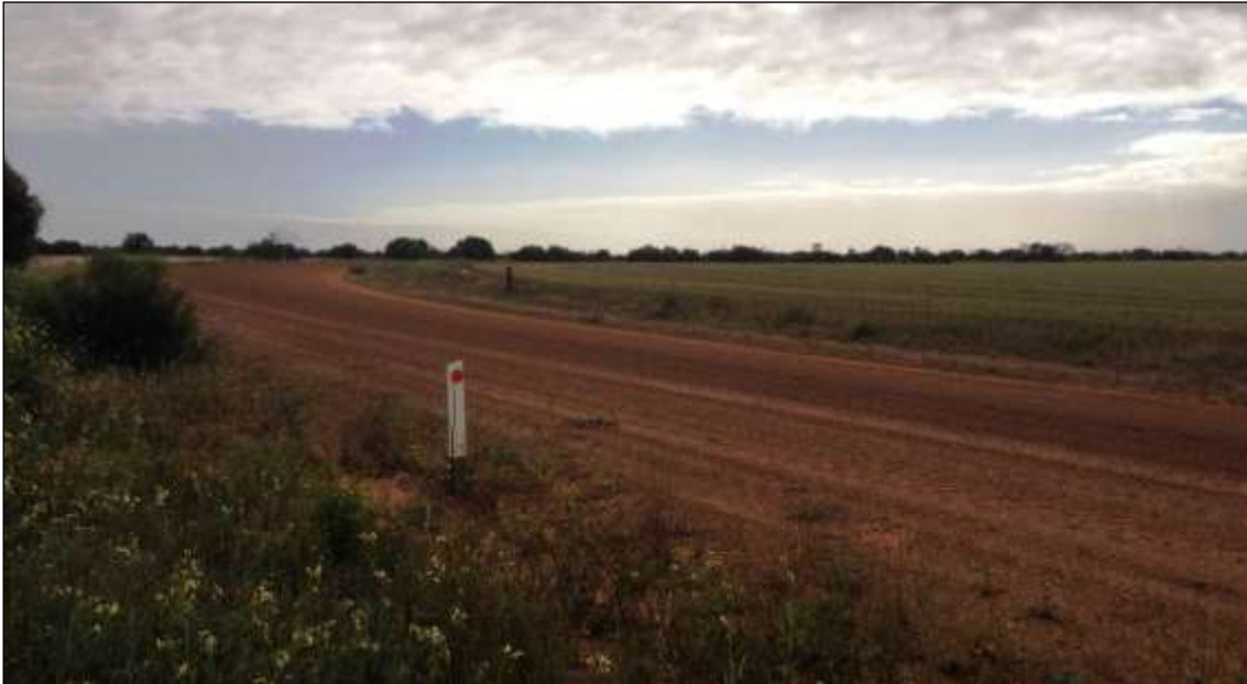
Figure 7 – View of East Nabawa Road Bend 4 looking north-east
