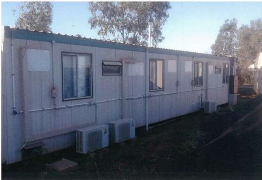
Below: View of rear of relocated building (all exterior wiring would be concealed behind new colorbond or weathertex cladding) this is proposed to be the northern elevation on Lot 18
