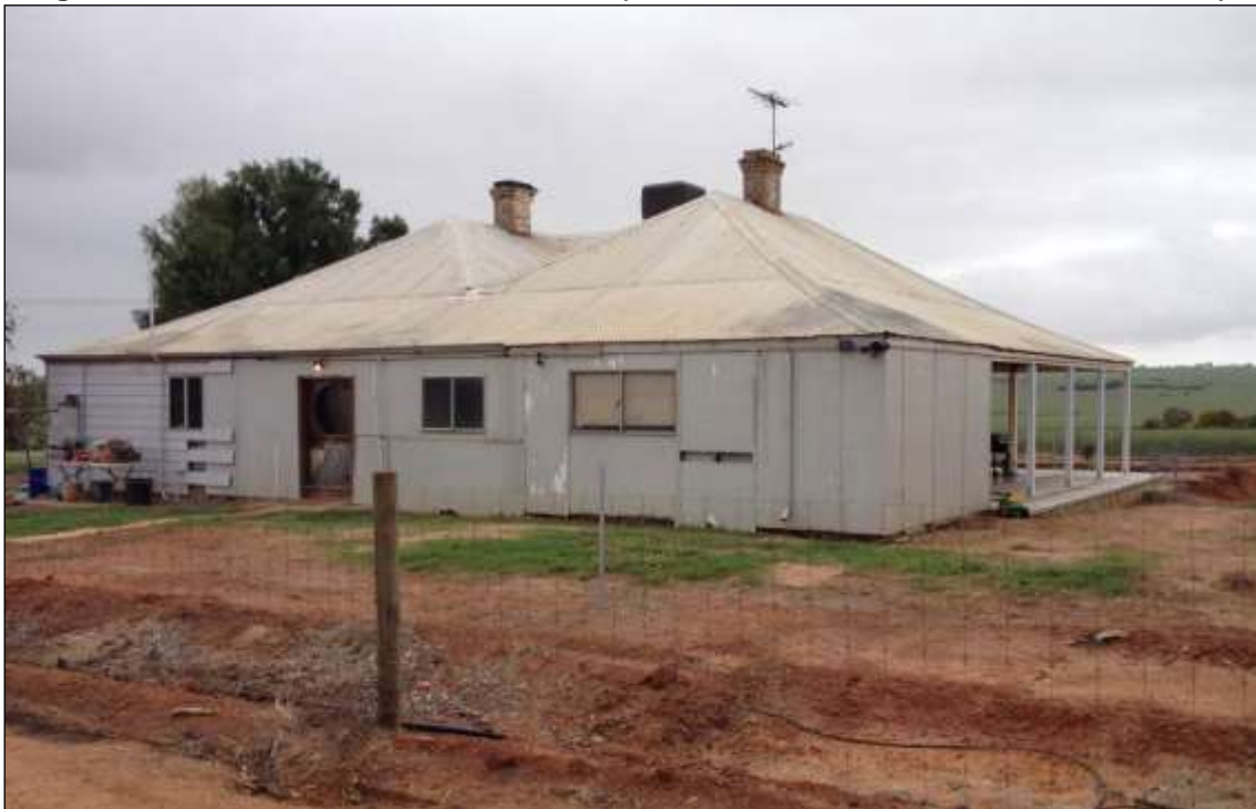
Figure 6 – Western elevation of residence (weatherboard extension to be demolished)
