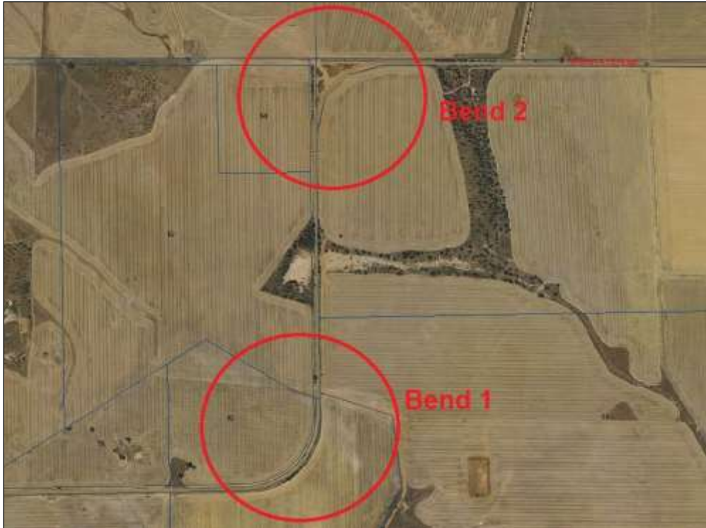
Figure 2 – Aerial Photograph of East Nabawa Road Bends 1 & 2
