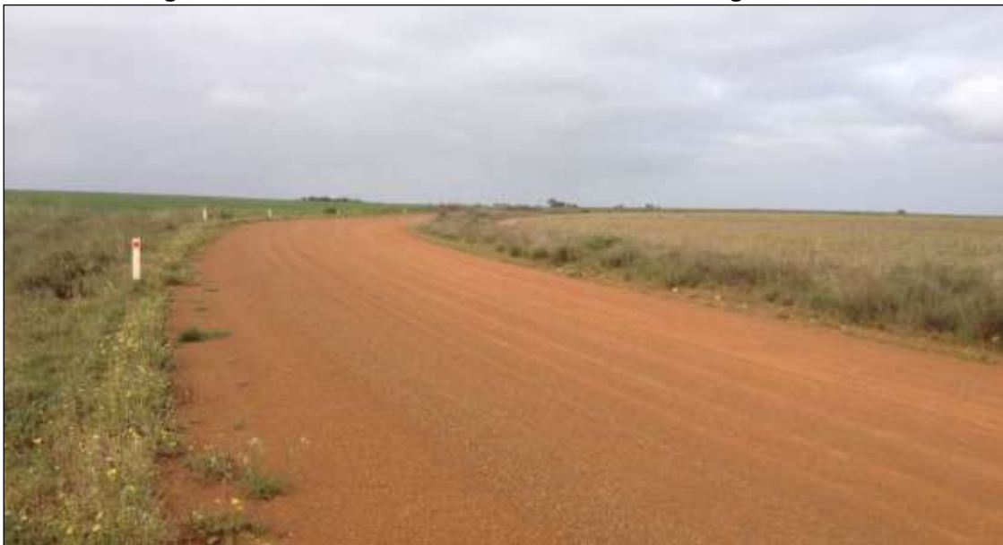
Figure 4 – View of East Nabawa Road Bend 1 looking north-east
