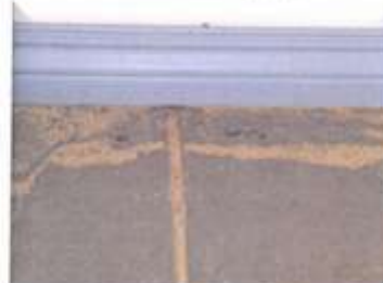
Tennis Club inside floor – insect and white ant issues due to building seal problem
