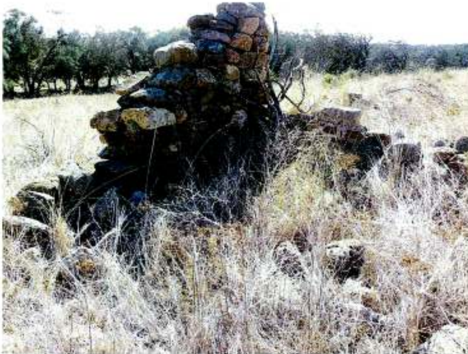
P06358 Stone dwelling (ruin), Howatharra View looking northeast showing the 'interior' of the north wall remains. L Gray 15 April 2010.
