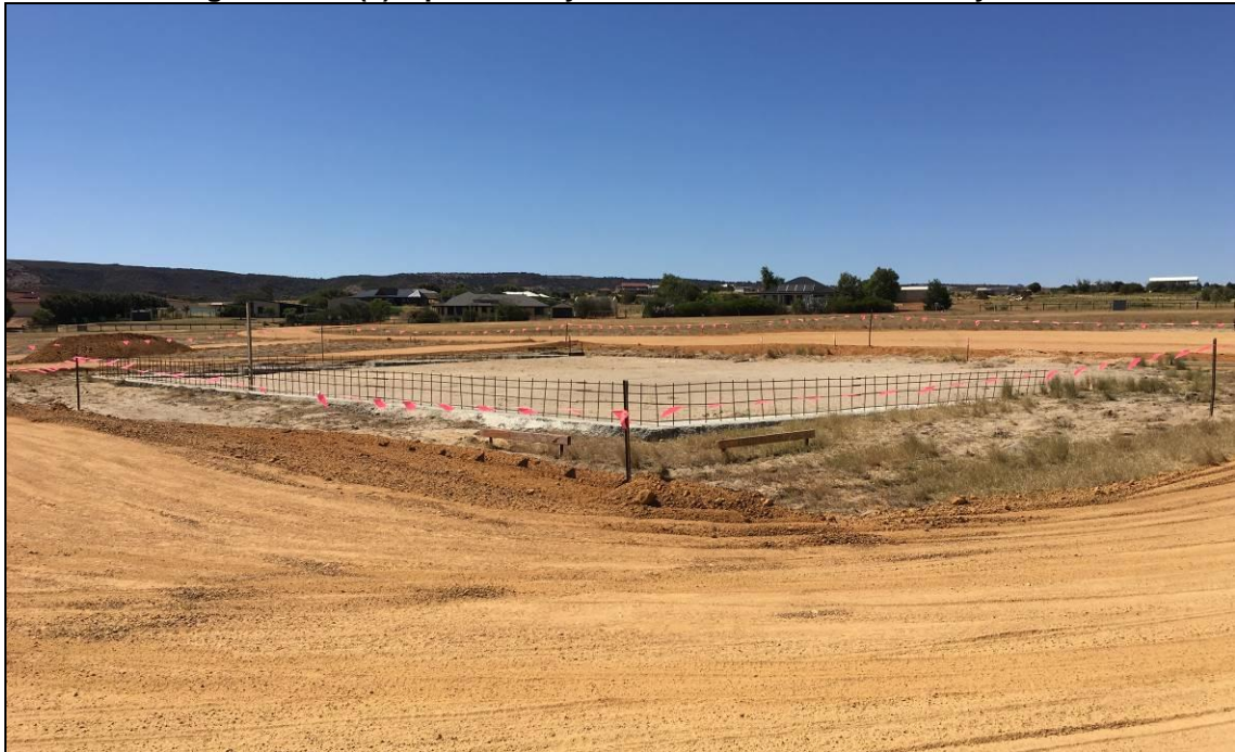
Figure 10.1.3(c) – preliminary access works at Bill Hemsley Park
