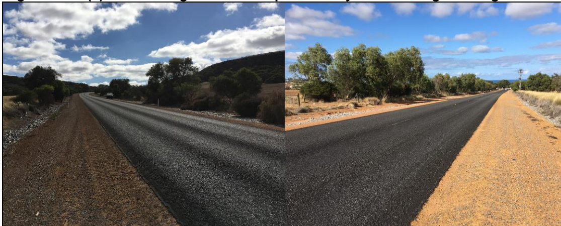
Figure 10.1.2(d) – view along Lot 1455 Chapman Valley Road frontage looking east/west
