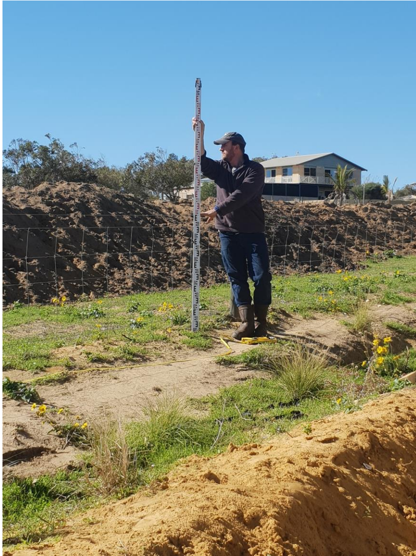
Lower Hand shows side fence height, highlighting pad height above neighbouring fence
