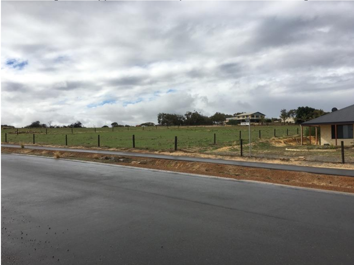
Figure 10.1.1(c) – View of Lot 121 prior to earthworks commencing
