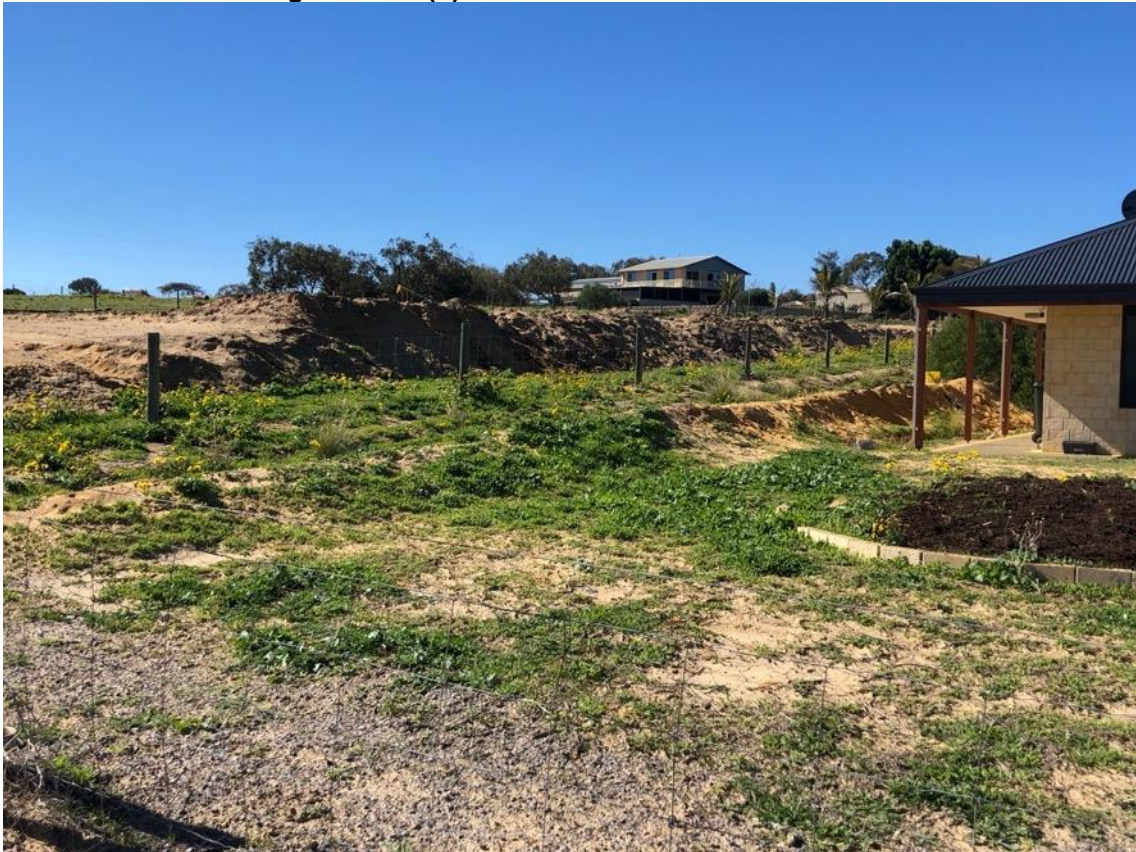
Figure 10.1.1(d) – Present earthwork level onsite
