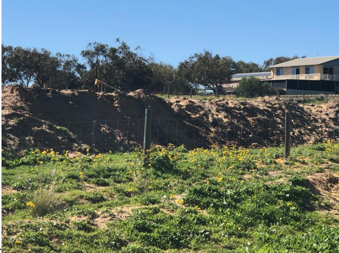
Figure 10.1.1(e) – Marker and rope showing proposed fill height and slope of batter towards southern Neighbour
