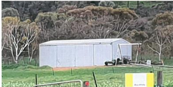
Figure 2: Existing Neighbouring Outbuilding
