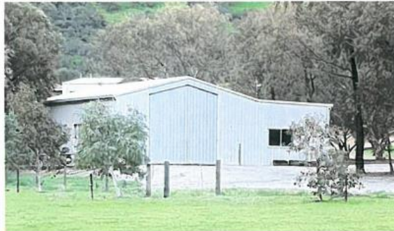
Figure 3: Existing Neighbouring Outbuilding
