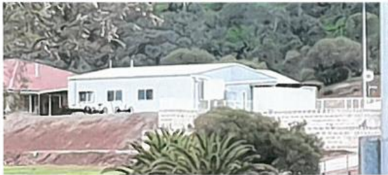
Figure 1: Existing Neighbouring Outbuilding
