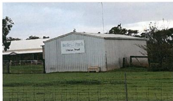
Figure 4: Existing Neighbouring Outbuilding
