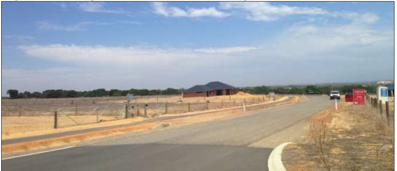
Figure 3 – View looking south from Dune Vista towards dwelling under construction on Lot 118
