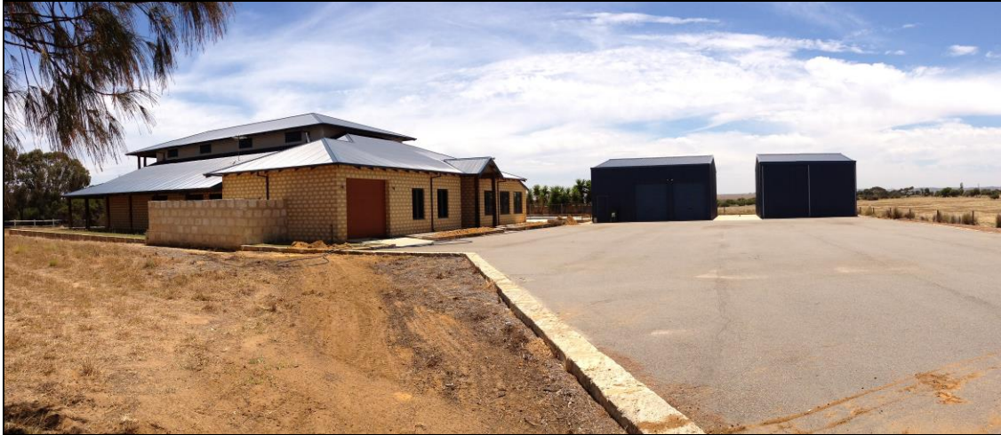
Figure 10.1.2(d) – View of Lot 50 from Eliza Shaw Drive following unauthorised works
