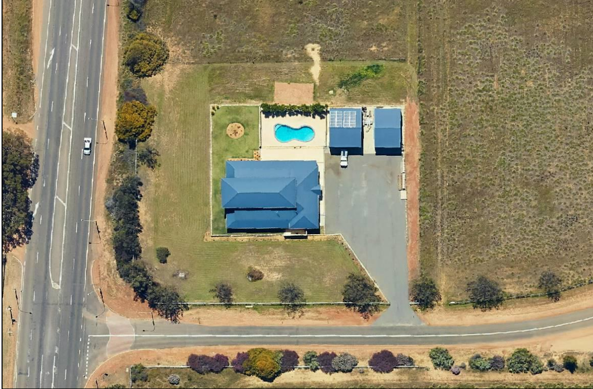
Figure 10.1.2(b) – Aerial photo of 5 (Lot 50) Eliza Shaw Drive prior to unauthorised works
