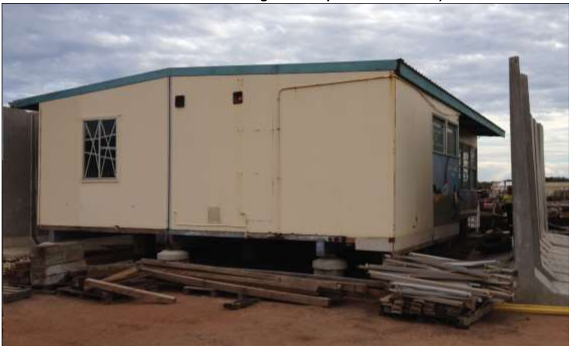
Figure 9.1.1(c) – View of relocatable building in its current Webberton location (this is proposed to become the eastern facing elevation and would have a 66.5m 2 gabled carport attached to it)
