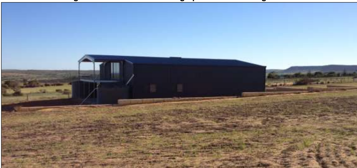
Figure 3 – View of outbuilding upon Lot 93 looking north
