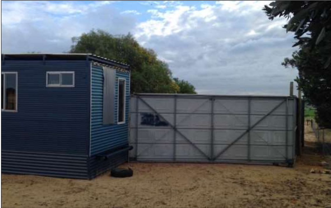
Figure 5 – View of outbuilding upon Lot 18 looking north, illustrating 5m setback
