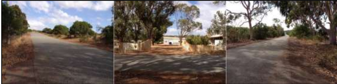
Figure 3 – View of entrance to business and Nanson-Howatharra Road approaches
