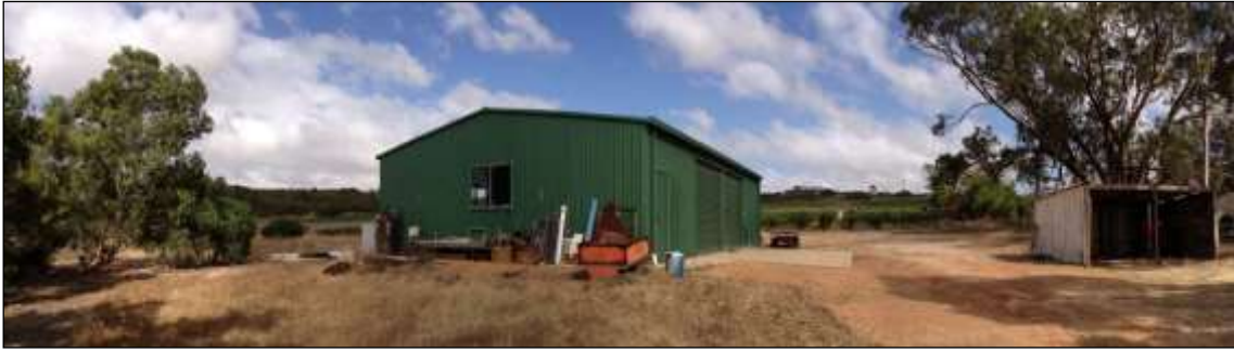
Figure 5 – View of Shed to be converted to micro-distillery, tasting and sales area
