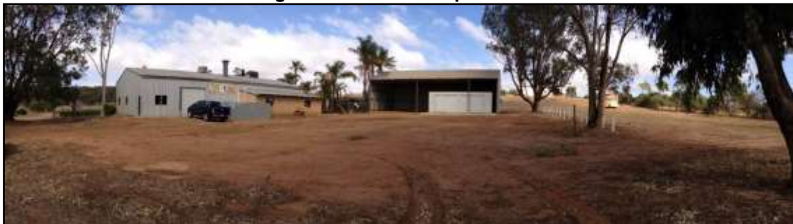
Figure 4 – View of car park area
