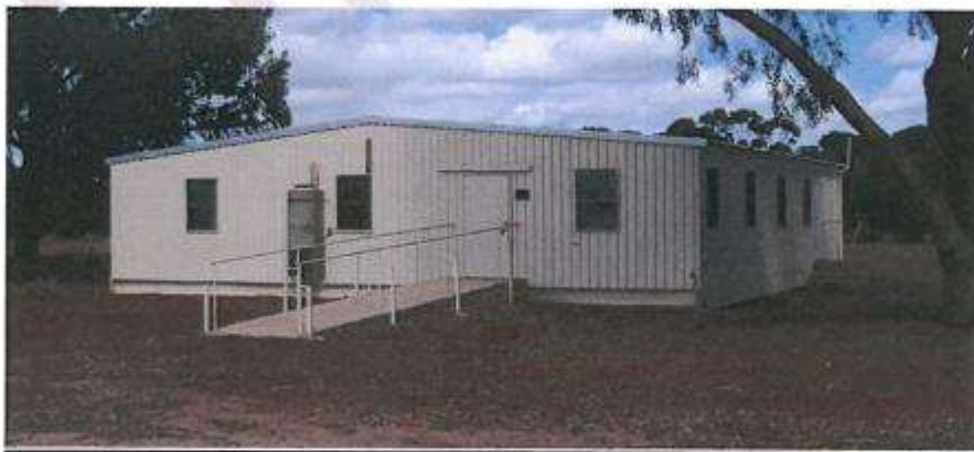
Transportable Building at Showgrounds at Nanson, looking from the East
