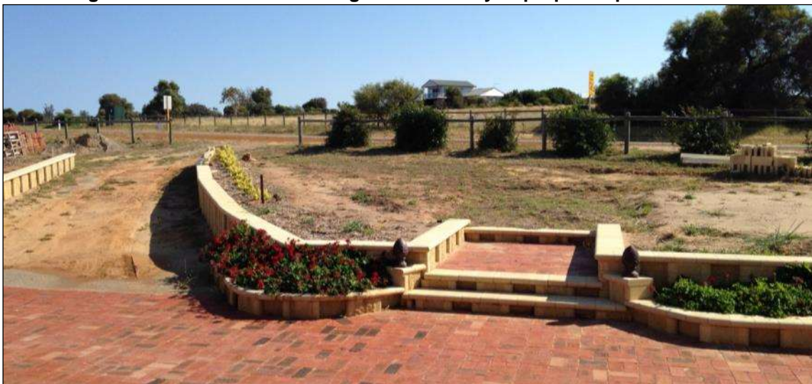
Figure 5 – View of stairs leading from driveway to proposed patio location
