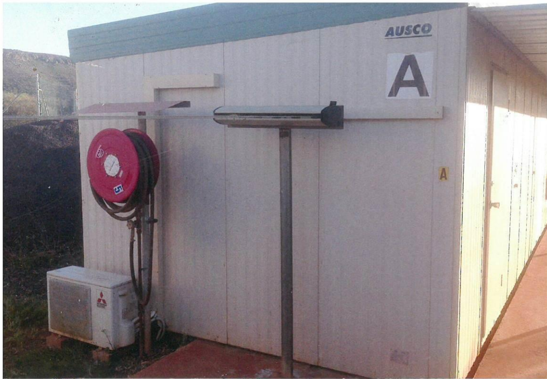
Above: View of side of relocated building (existing hose reel would be removed) this is proposed to be the western elevation on Lot 18
