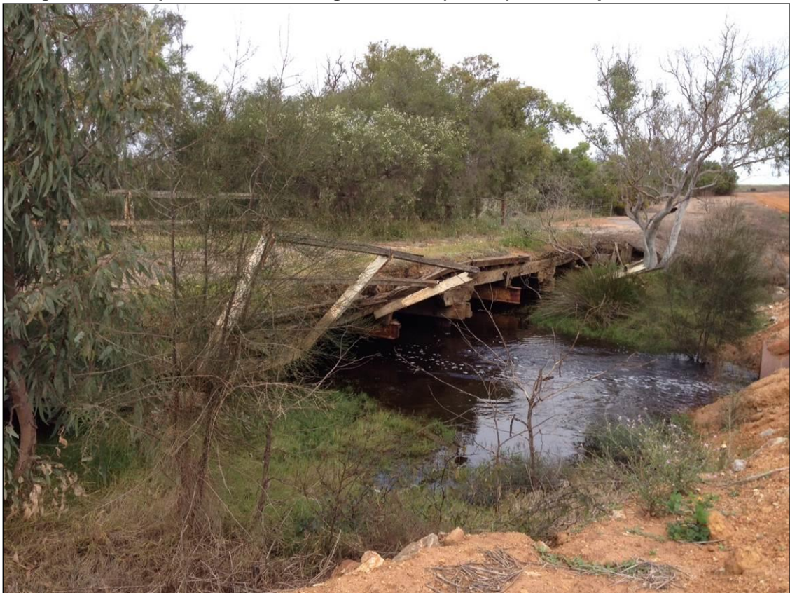
Figure 13 - Chapman River crossing on closed (former) East Chapman Road reserve
