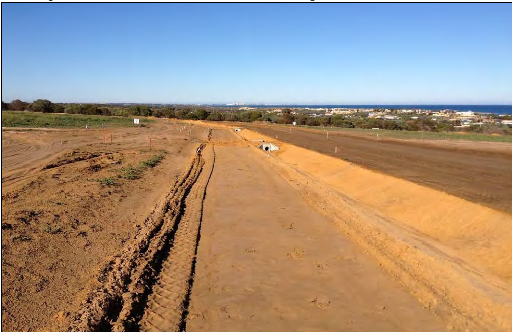
Figure 3 – View from centre of Lot 2 looking south towards Geraldton
