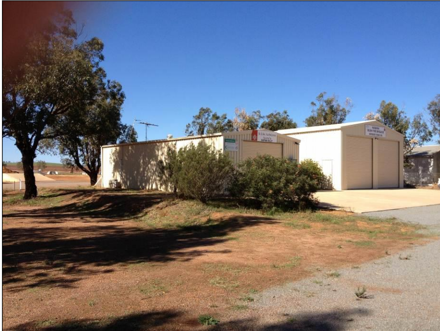
Figure 2 – Photograph of Chapman Valley Ambulance Sub Centre looking south-east
