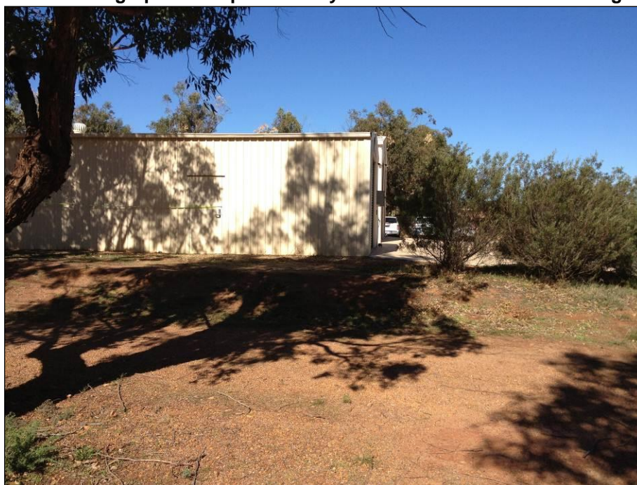
Figure 4 – Photograph of Chapman Valley Ambulance Sub Centre looking south
