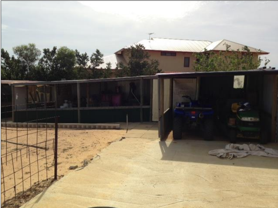
Figure 4 – View of existing outbuilding structures to rear of residence upon Lot 211
