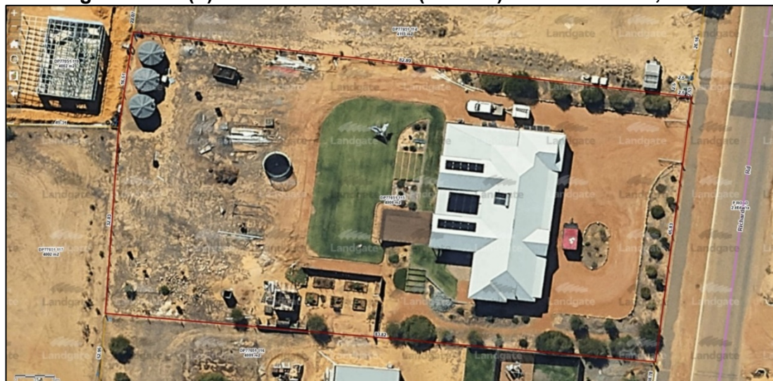
Figure 10.1.1(b) – Aerial Photo of 27 (Lot 115) Richards Road, Buller
