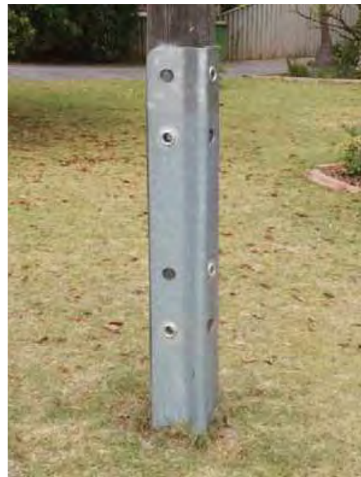
Figure 5 – Typical reinforcement of timber poles with steel supports
