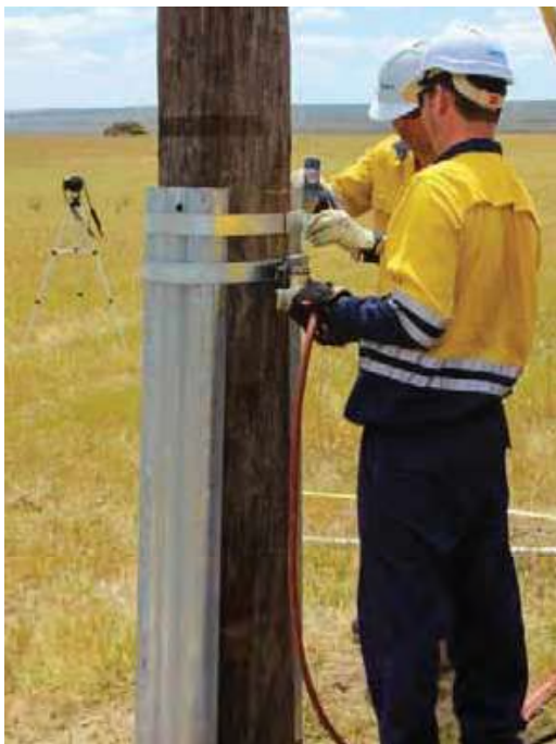
Figure 5 – Typical reinforcement of timber poles with steel supports
